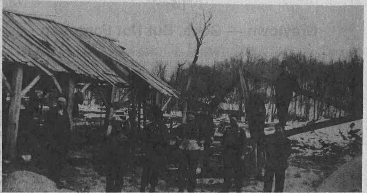
A sawmill crew in 1916 poses for a picture near a shed. These men worked for Chester B. Thatcher in the Graytown sawmill.
